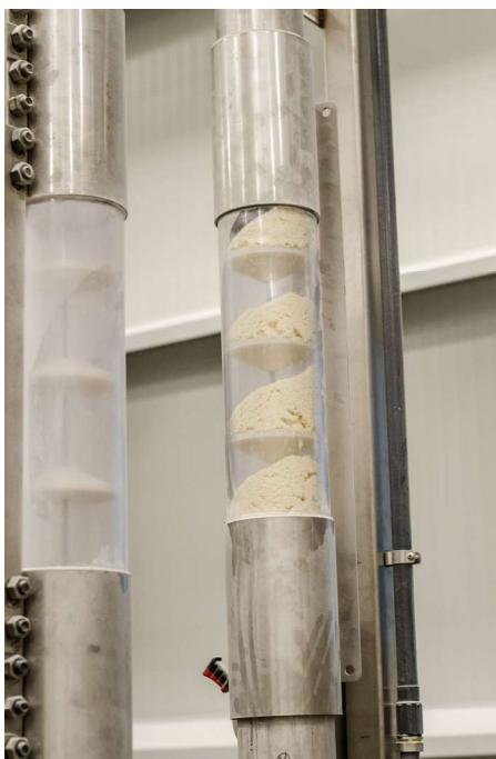
Transportation of finished product to packaging or loading is through a Cablevey system.
