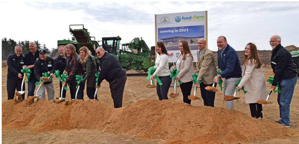
Farming for the Future Foundation board members, along with Wisconsin Secretary of Agriculture Randy Romanski and Chris Roth, president and CEO of Reinke Manufacturing Company, broke ground on the Food + Farm Exploration Center, April 29, in Plover, Wisconsin. From left to right are Paul Palmbly; Richard Okray; Tamas Houlihan; Les Dobbe; Andy Diercks; Jordan Lamb; Richard Pavelski; Michelle Peariso; Alicia Pavelski; Roth; Sec. Romanski; Candise Miller; and Gregg Hansel.
