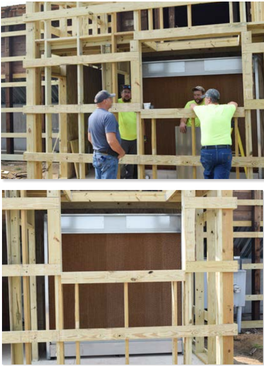
From left to right, Eugene Mancl, Tyler Jacoby, Daniel Hafstad, and Greg Johnson of Ron's Refrigeration discuss the new Humidicell recently installed in an Okray Family Farms potato storage building as part of a complete remodel. The building was originally built with downflow systems and louvers for intake air, which fell out of favor years ago. As part of the revamp, three new systems feed the same building and include state-of-the-art control panels (IVI Sentinels), Humidicells, refrigeration, and thermal doors for intake air, along with a custom-built high-pressure fogging system for supplemental humidity.
