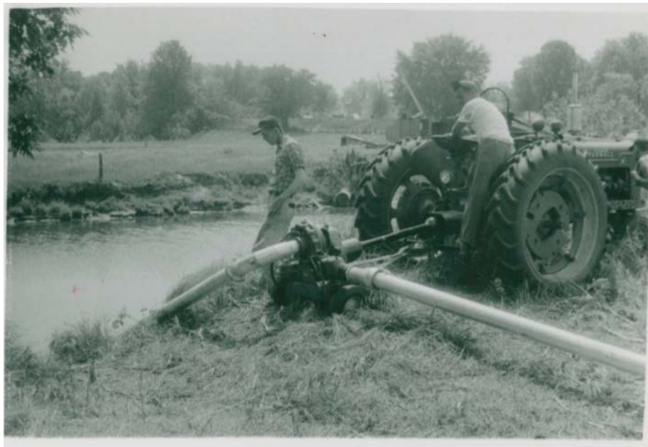
Above: In this early Roberts Irrigation photo from when Hal Roberts ran the operation, a tractor is used to run a pump and pull irrigation water from a local source.
